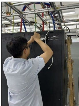
Install the MOS
